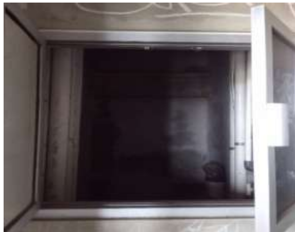
Picture 2 : Elevator shaft
