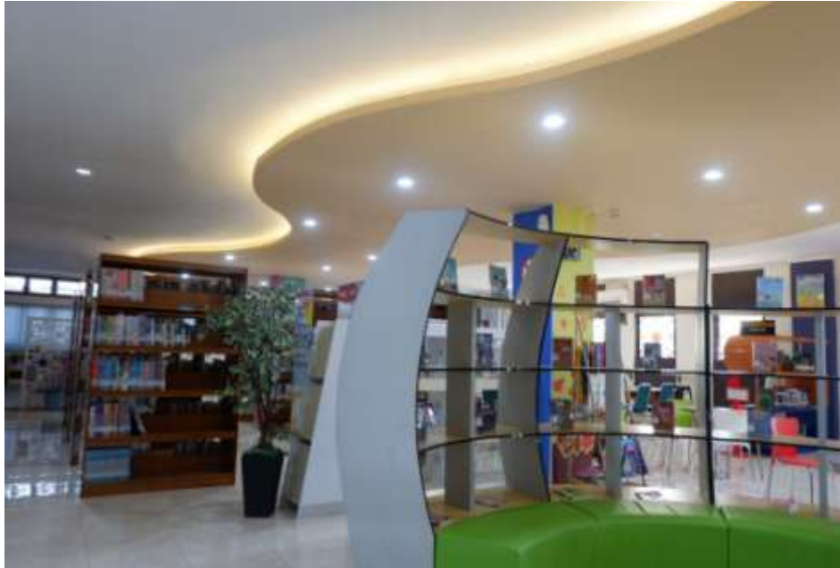
Picture 8 : Condition of Ceiling Source : Researcher's Documentation, 2023
