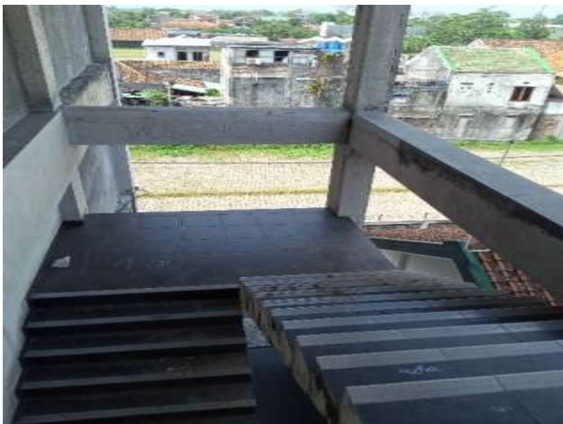
Picture 4 : Emergency Stairs Source : Researcher's Documentation, 2023
