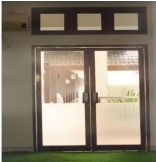
Picture 7: Library Emergency Exit Source : Researcher's Documentation, 2023
