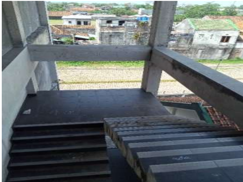
Picture 4 : Emergency Stairs Source : Researcher's Documentation, 2023
